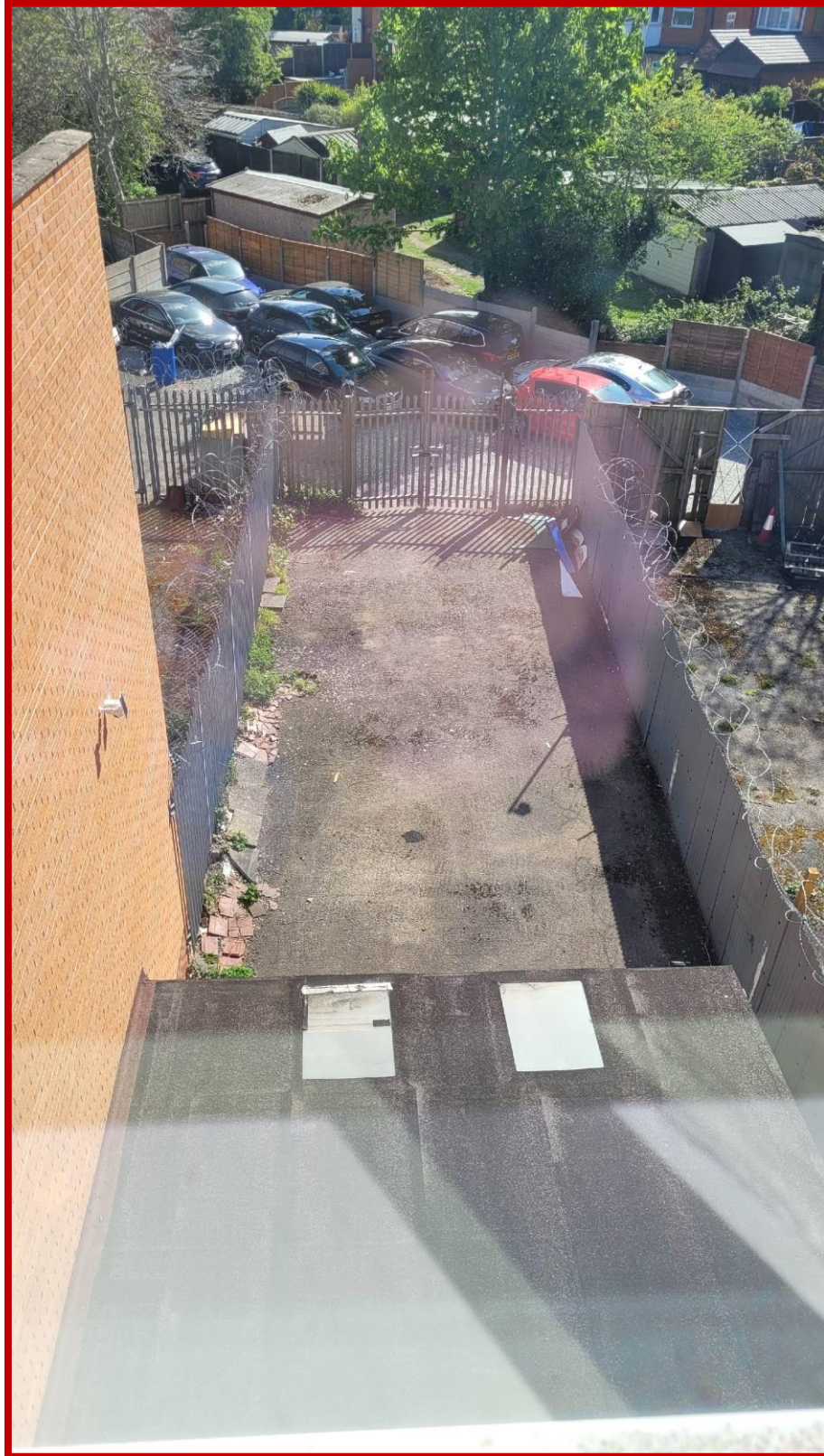
Rear Yard & Car Park
